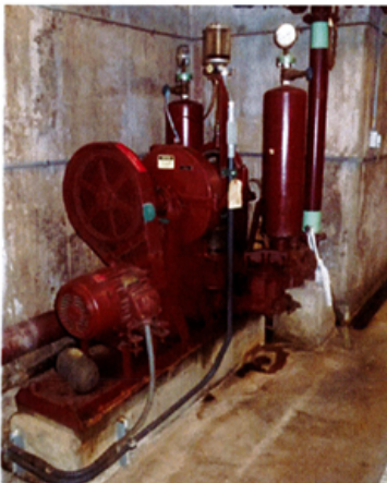
Replace Primary Scum Pump and Remove Secondary Scum Pump
