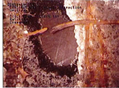
Photo of failed roadway from inside the culvert structure
