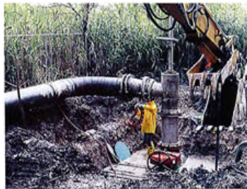
Emergency Repair bypass system.
