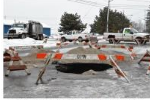
Pipe deterioration caused by infiltration under Milton Ave – sink hole
