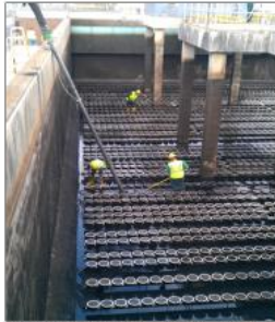
Metro WWTP Aeration Cleaning. Staff from Maintenance, Flow Control and Operations collaborated in an aeration tank cleaning project. Aeration discs are later chemically cleaned to reduce plant operational energy costs. Similar work currently ongoing at Meadowbrook Limestone.
