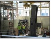
Metro Screen &amp; Grit: WEP completes the replacement of screens at the headworks of the Metro plant. Teamwork and coordination toward critical replacement while flow always continues.
