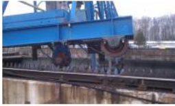
Even the best maintenance can't always keep a Reagan era traveling bridge on the rails! Current construction at Oak Orchard will replace the traveling bridge.
