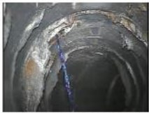
WEP Flow Control – maintaining &amp; televising sewers, an example of an illicit discharge to a storm sewer. WEP protects the environment.
